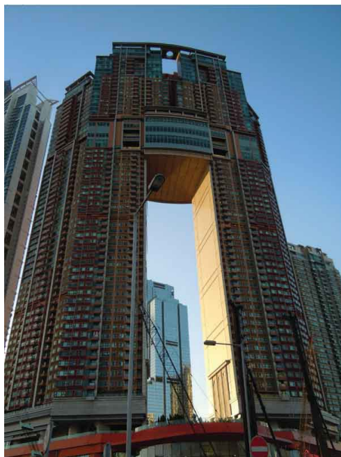
Feng shui building in Hong Kong (Hong Kong Island).
