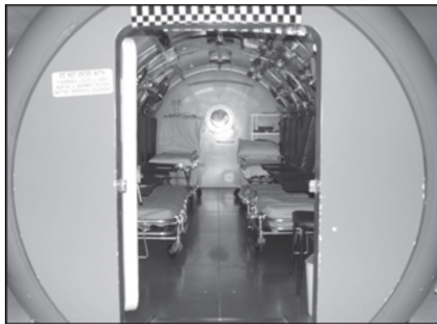
FIGURE 7. This figure depicts the inside of a typical multiplace chamber, the chamber featured in Figure 8 . The main lock or treatment lock is seen with four stretchers in place.
